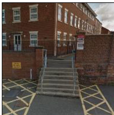
Photo (Eastbound): Stepped access from Station Road to Queen Street/Launder Terrace
