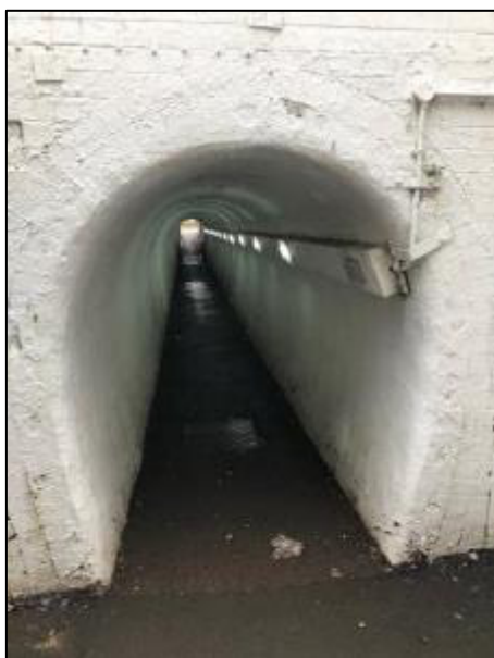
Photo (Westbound): Subway running from Station Road to Huntingtower Road.
