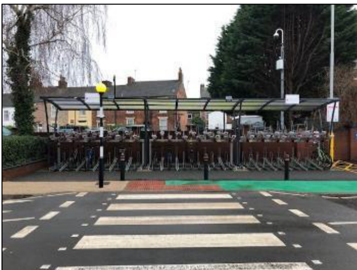
Photo (Eastbound): Cycle parking opposite station entrance with zebra crossing.
